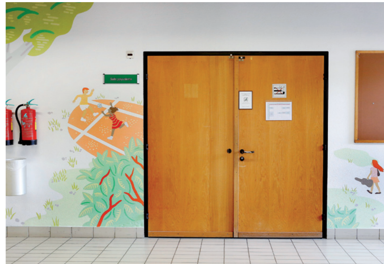
Exterior wall of the multipurpose room: scene illustrating the activities practiced
