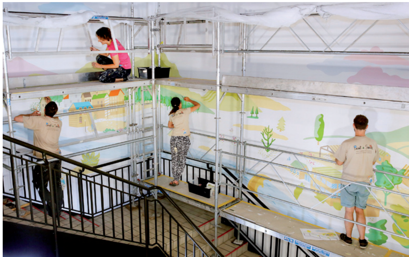
Stairs between the ground floor and the garden level: main scene of the project in progress
